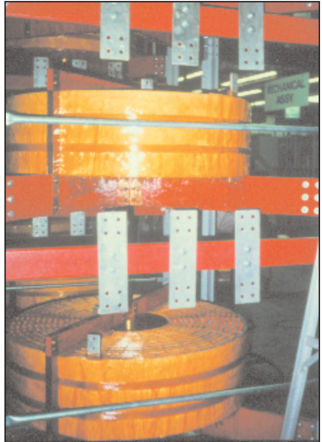
Figure 2. Terminal bars in this 5 kV reactor assembly are drilled for bolted attachment of multiple cable lugs. Uniform loading and heating of all connections requires uniform tightening of all hardware.
