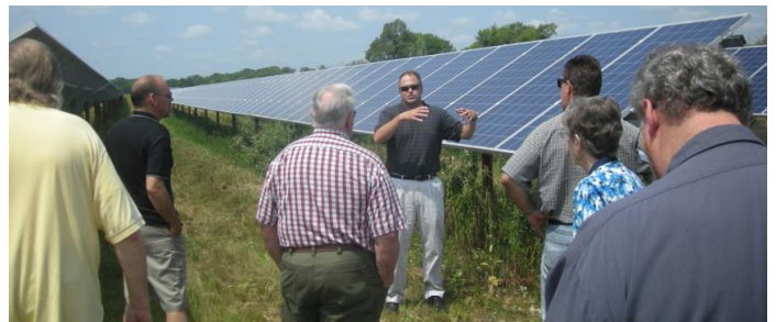
Brent Anderson of Wanxiang describes the construction and operation of their 3 MW, 10,000 panel solar farm near the Rockford airport.
