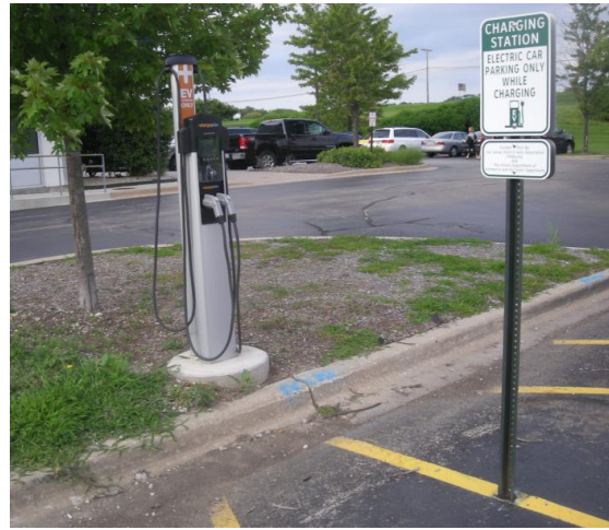
Chargepoint Charger and sign
