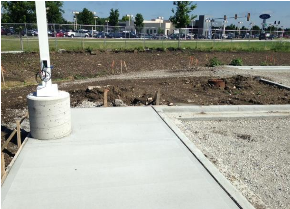
Sidewalk just poured at CCC 7/10/2014... almost ready for charger installation!
