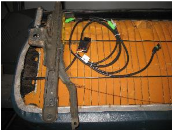
Wiring harness installed underneath seat.
