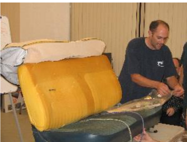
Cover peeled back, prepare to install heater. Cut out some foam to inlay thermostat.
