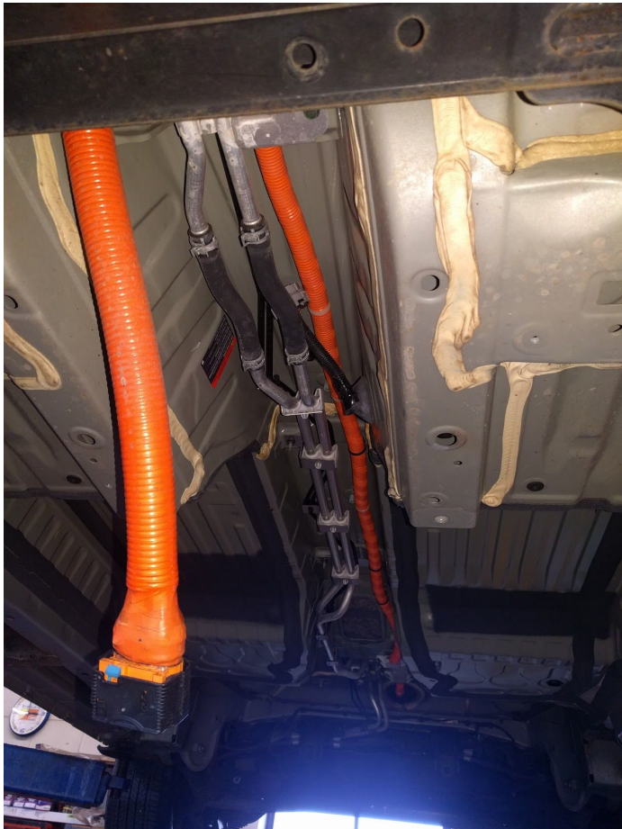
The high-voltage and control wiring that neatly runs between the vehicle and battery pack is exposed once the battery pack is removed.
