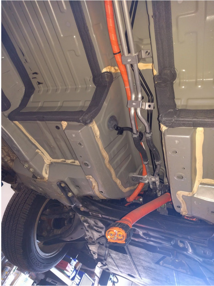
High-power and control wire connectors that were detached from the battery pack.
